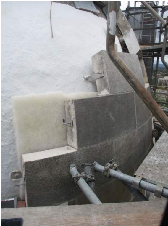
Figure 7. Dome restoration in progress
