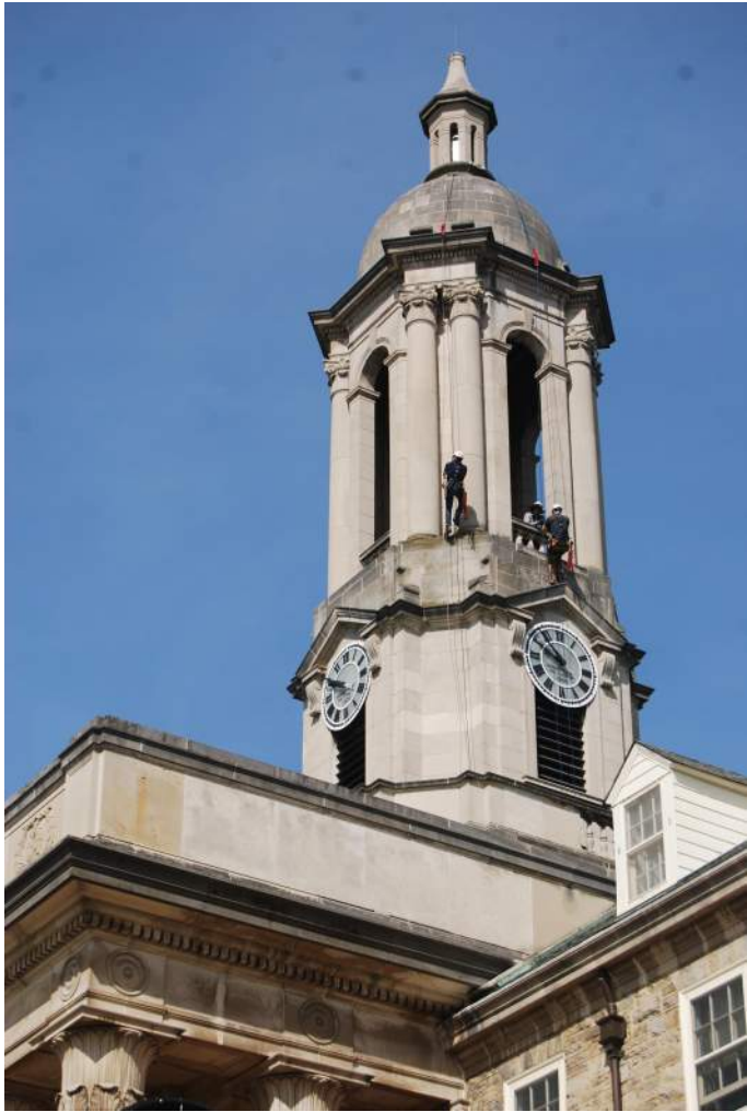
Figure 4. Industrial rope access survey of bell tower
