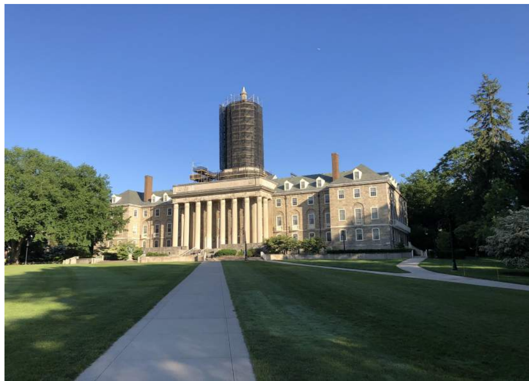
Figure 5. Bell tower encased in scaffolding
