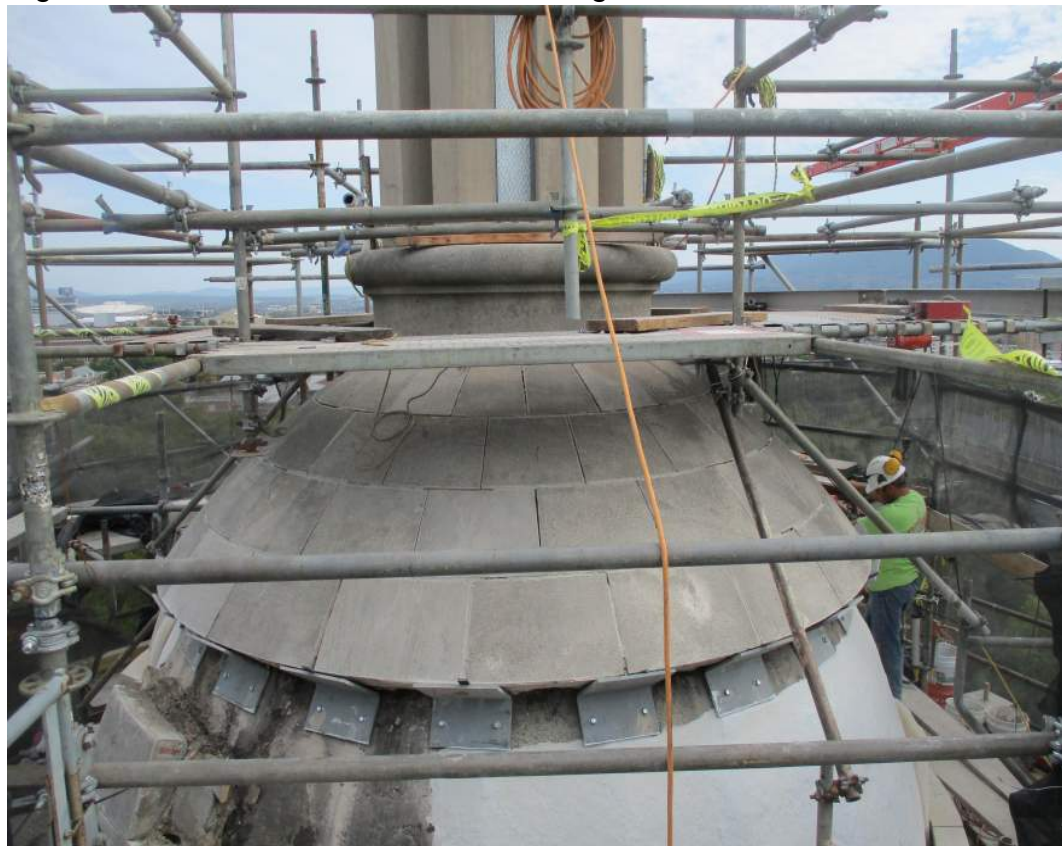
Figure 6. Limestone cladding removal and waterproofing in progress
