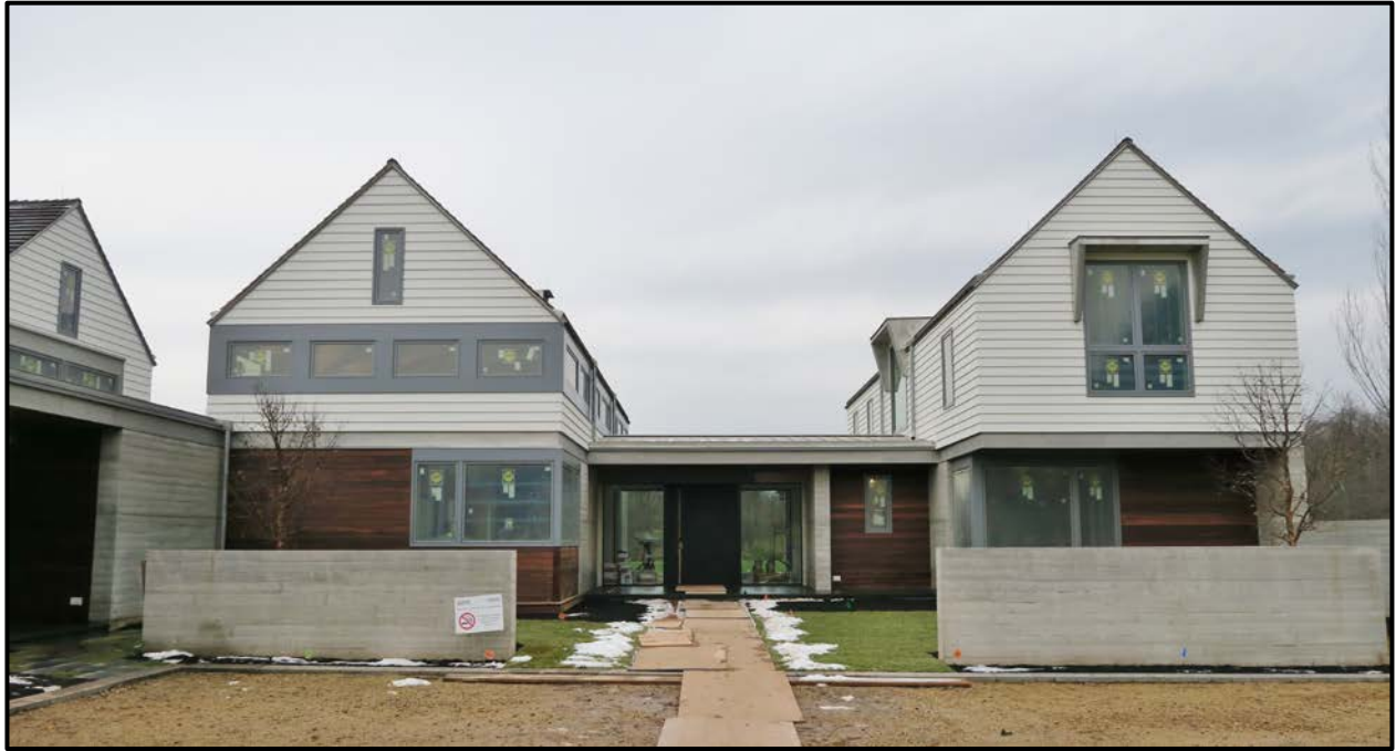
Photo of front of home: Two story kitchen/dining room/living room space on left, guest wing on right
