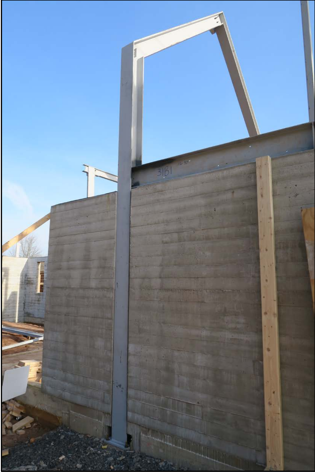
Construction photo of board-formed wall at great-room
