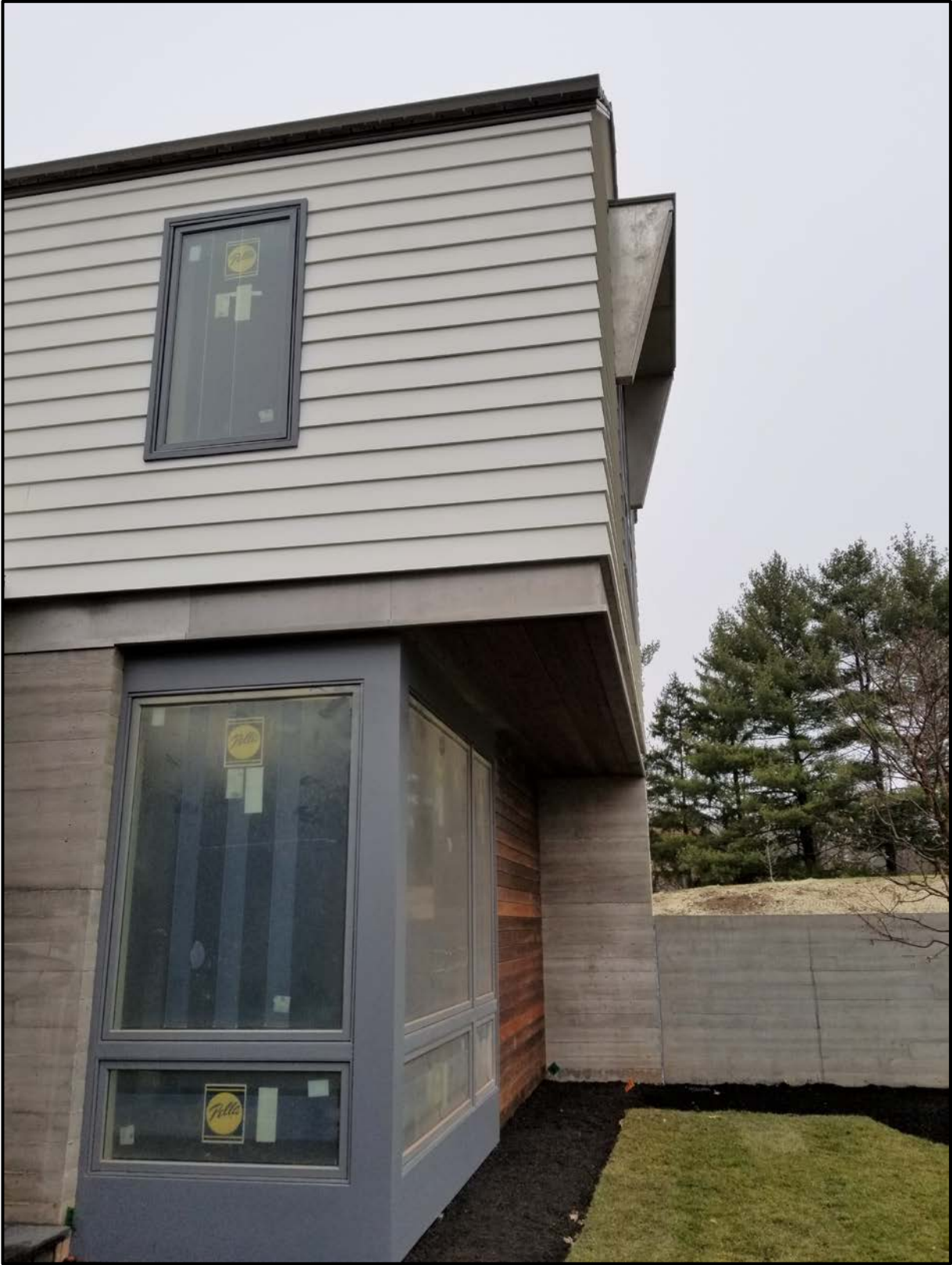
Photo of cantilevered second floor corner at guest wing
