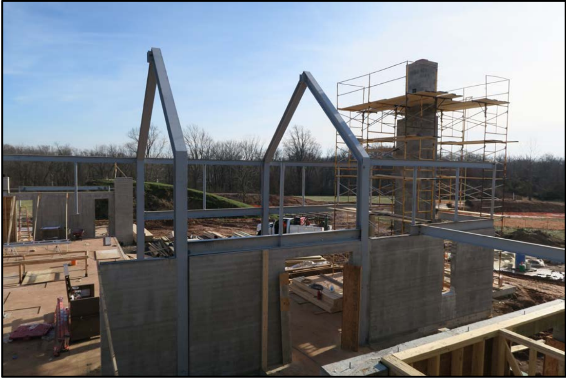
Construction photos of great room steel frames
