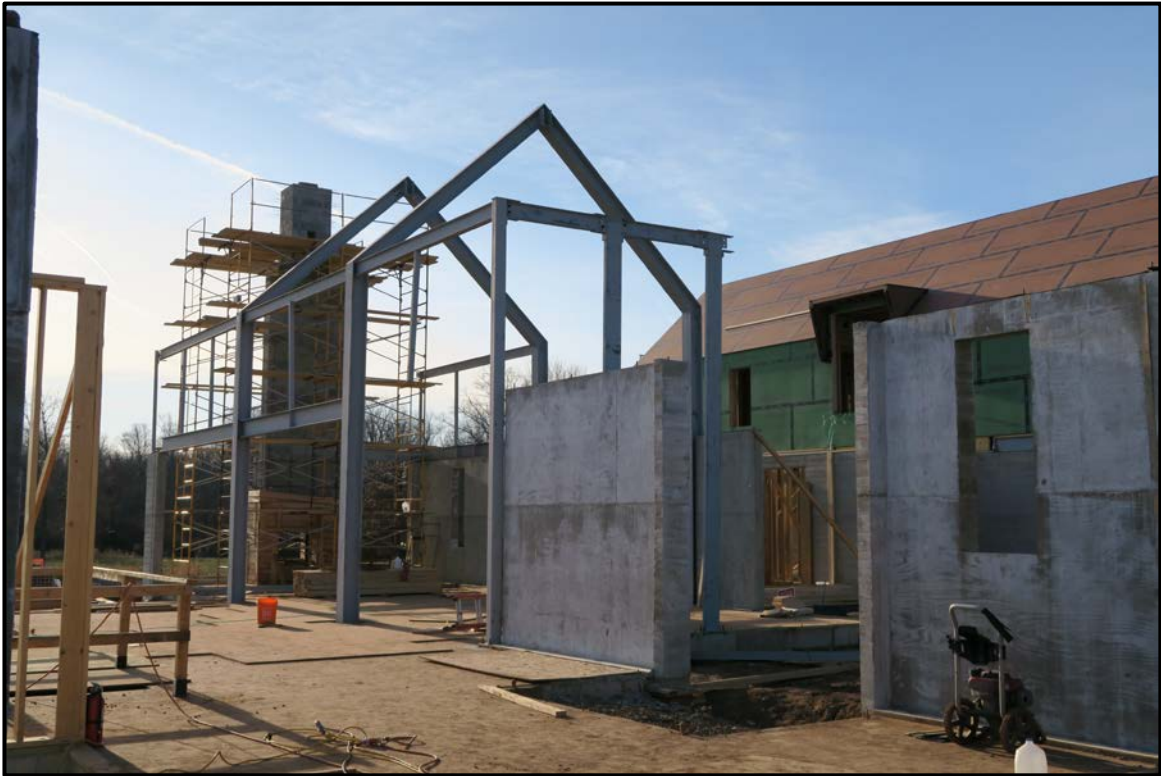
Construction photos of great room steel frames
