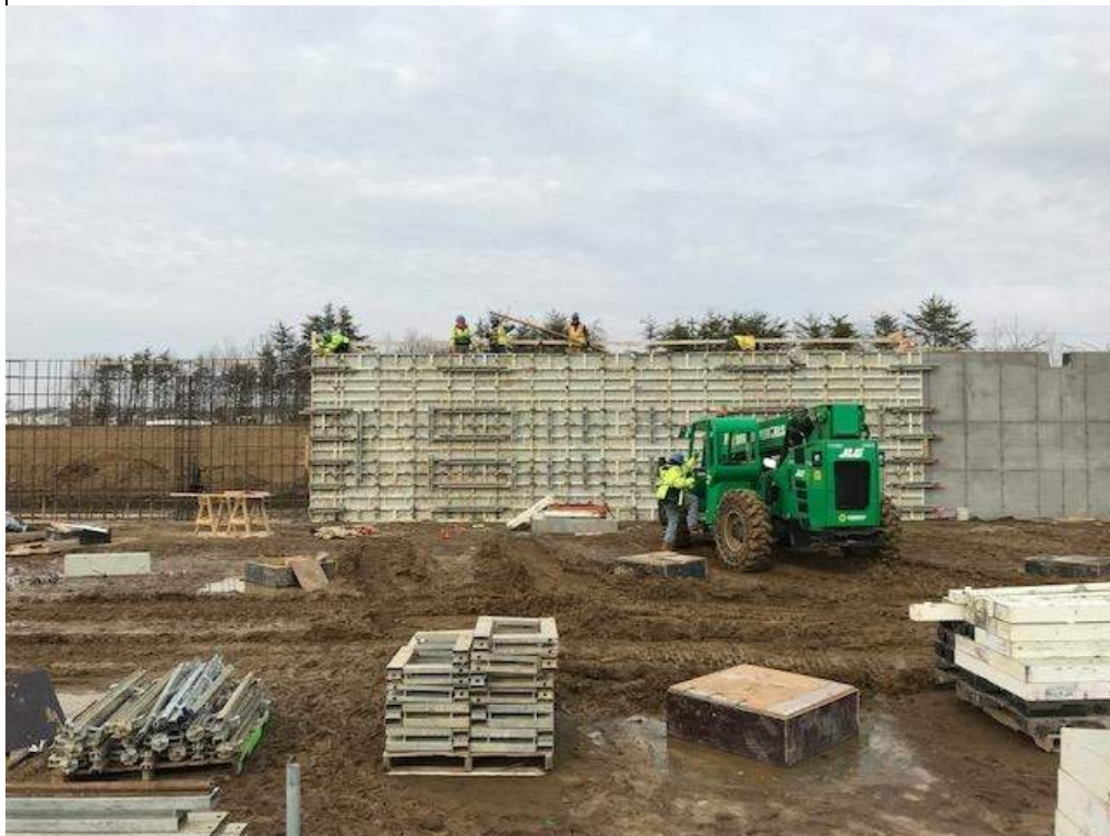
Above image: Drone photo of site taken while working on foundations. Below image: Forms being installed for cast in place concrete wall.
