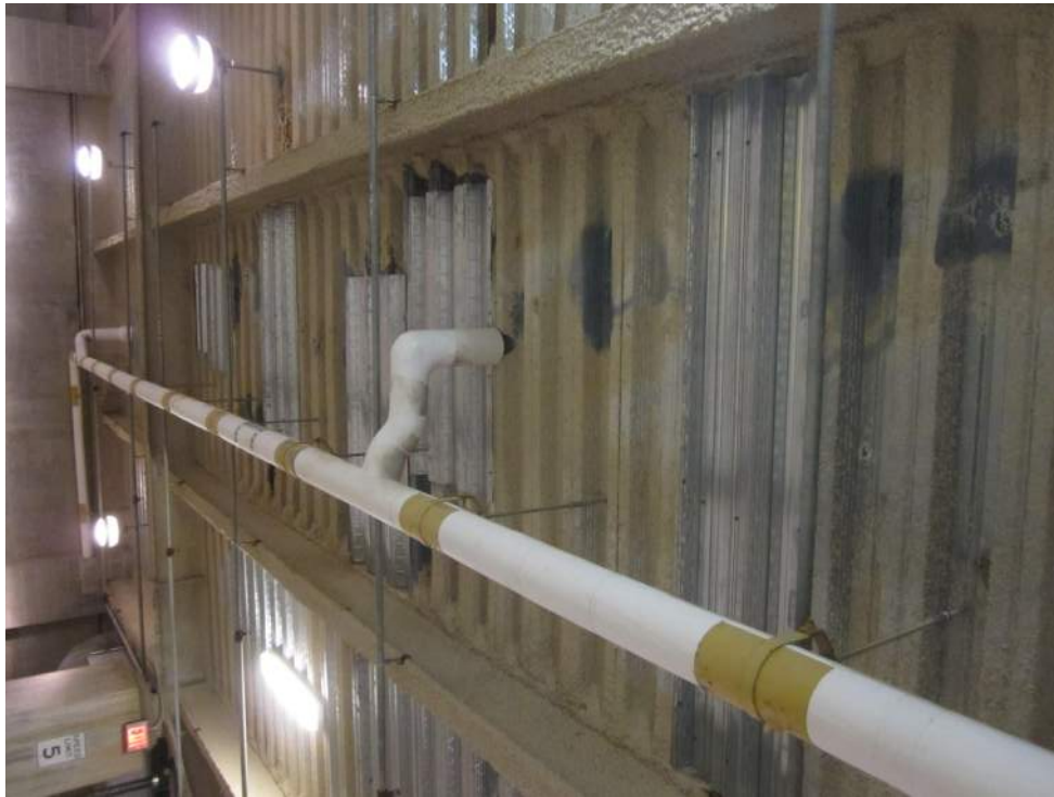
Figure 1. Supplemental decking added to supplement metal deck that corroded through.
