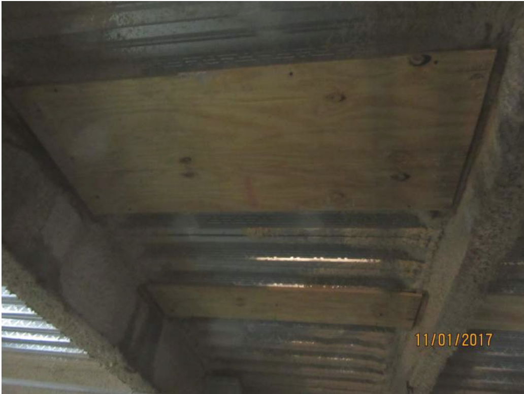
Figure 5. Formwork for isolated full-depth repairs.
