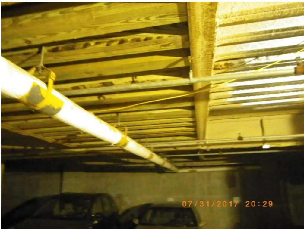
Figure 4. Supplemental shoring / work area support.
