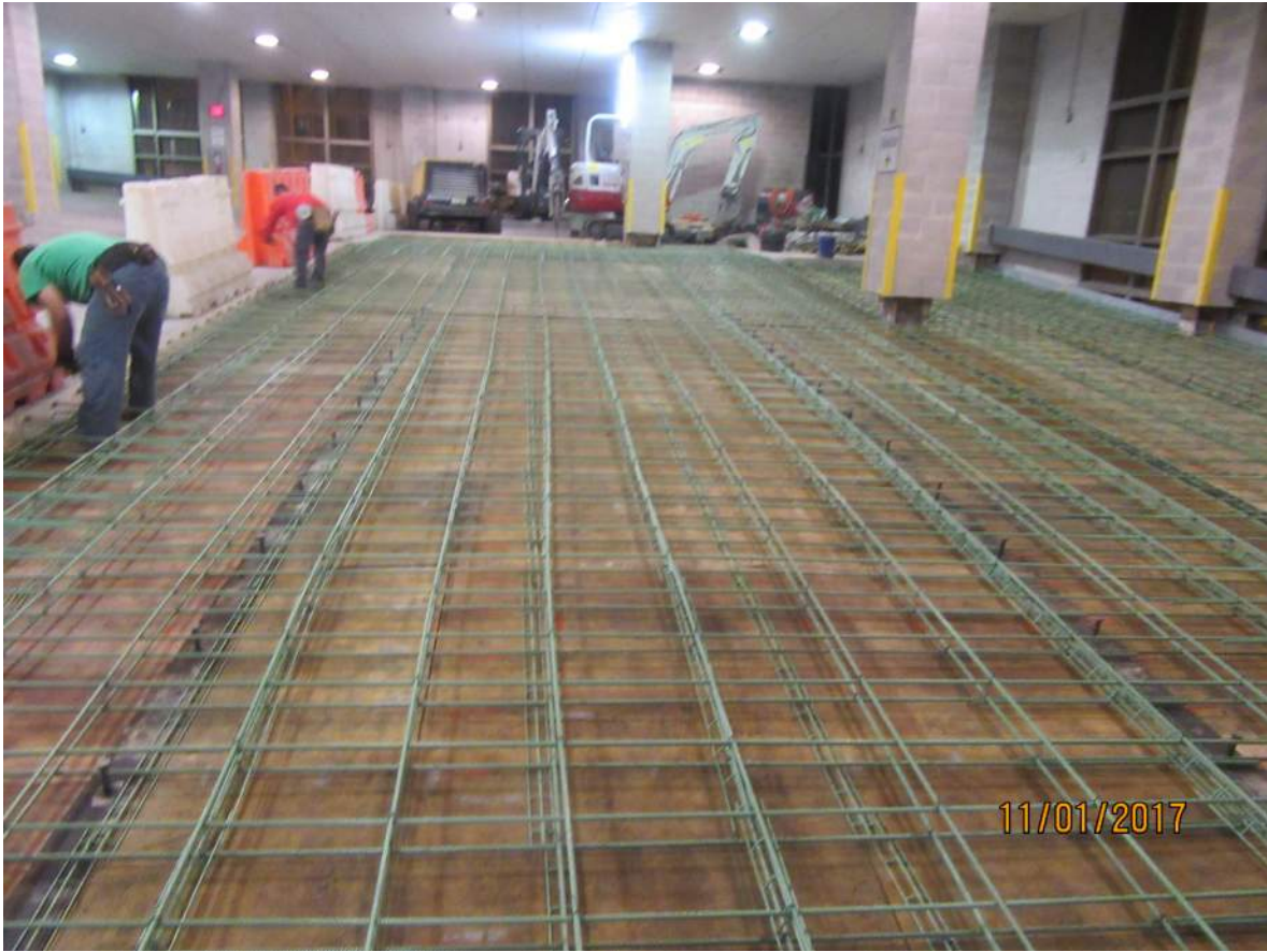
Figure 8. Deck reinforcement in place prior to concrete placement.
