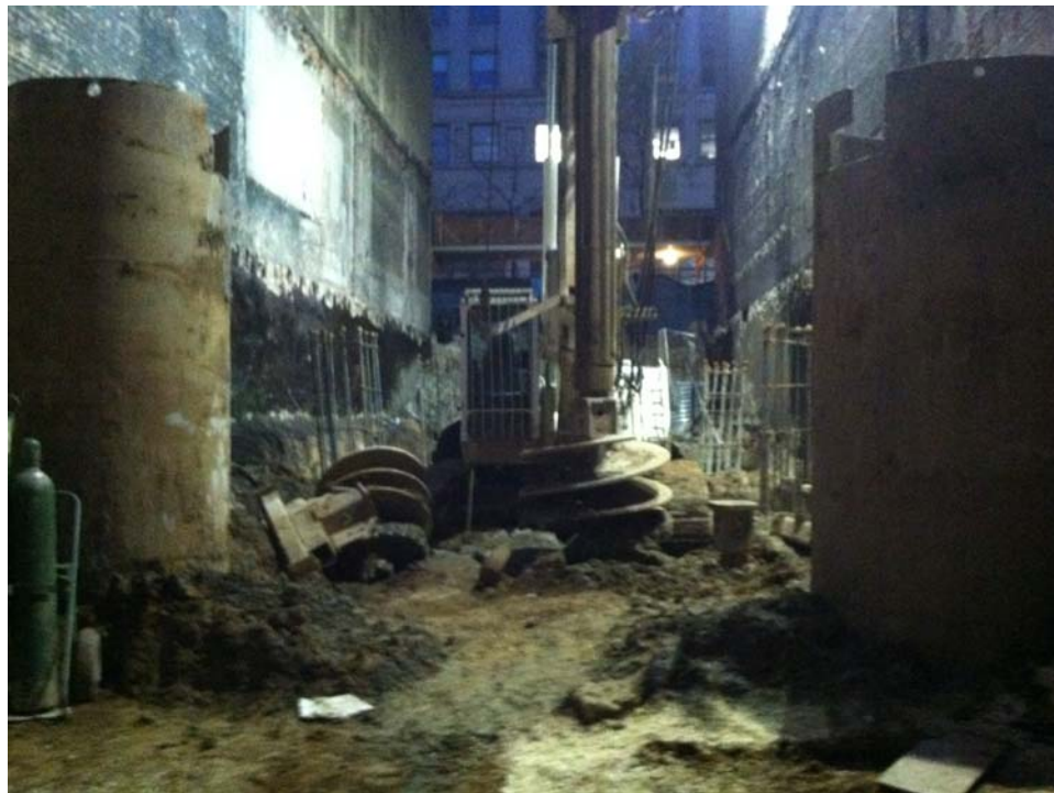
Caisson drilling rig at the bottom of the
